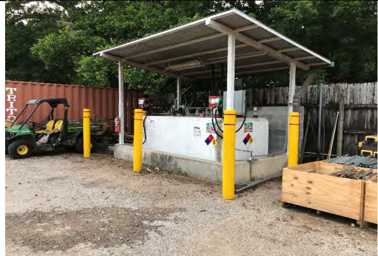
Photo 2: View of Unleaded Gasoline and Diesel fuel AST on the south side of the Maintenance Barn area. Facing southeast.
