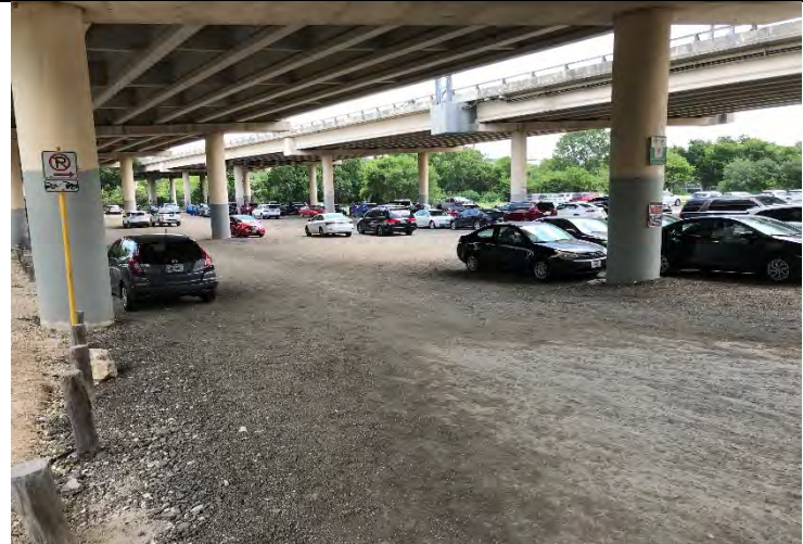
Photo 26: View of the asphalt paved parking area on the Butler Landfill cap beneath Mopac. Facing northeast.
