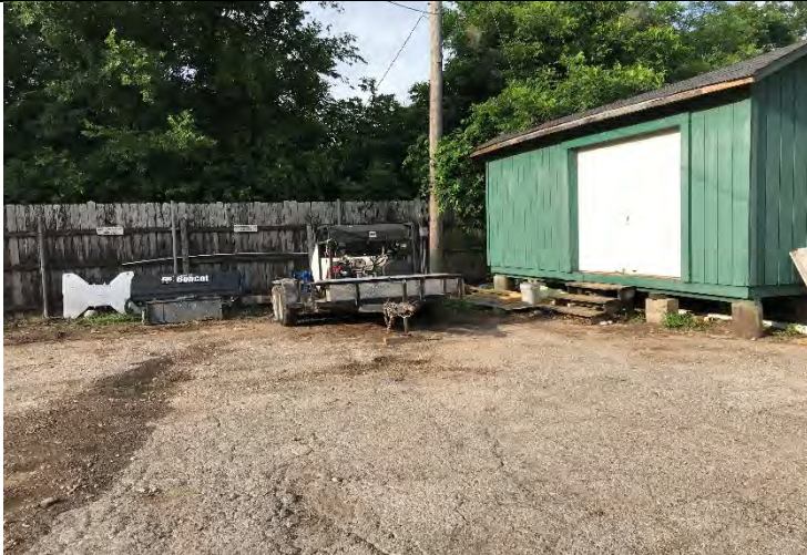
Photo 1: View of storage shed and former UST location in the southwest portion of the Maintenance Barn area. Facing south.
