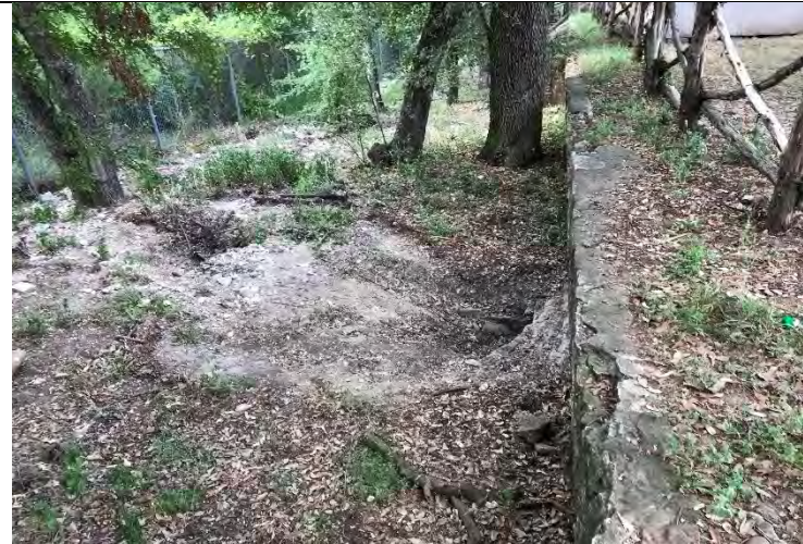
Photo 44: View of the storm water flow path beyond the outfall pictured in Photo 43. Facing south.
