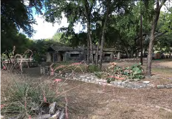
Photo 35: View of the Pistol Range rock building and retaining walls that show the grade elevation change between the former shooting area and the building. Facing southwest.
