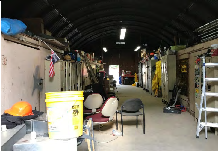
Photo 9: View of the interior of the Maintenance Barn. Facing west.
