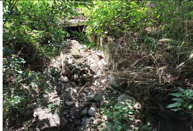
Photo 42: View of the inlet to the storm water conveyance at the northwest corner of the Pistol Range. The inlet receives storm water from the area to the north and northwest of the Pistol and Skeet ranges. Facing south.
