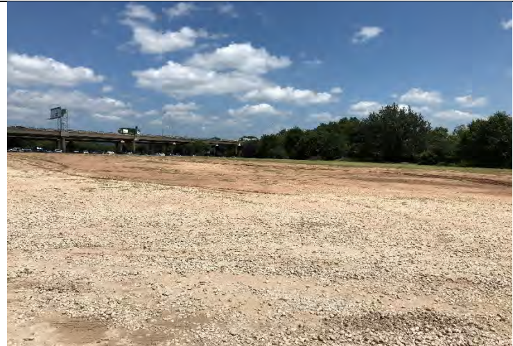
Photo 24: View of the transition from gravel to soil in the central portion of the Butler Landfill cap. Facing north-northwest.
