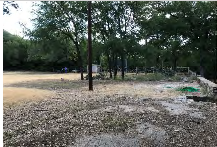
Photo 28: View of former covered shooting area in southern portion of the Pistol Range. Facing east.
